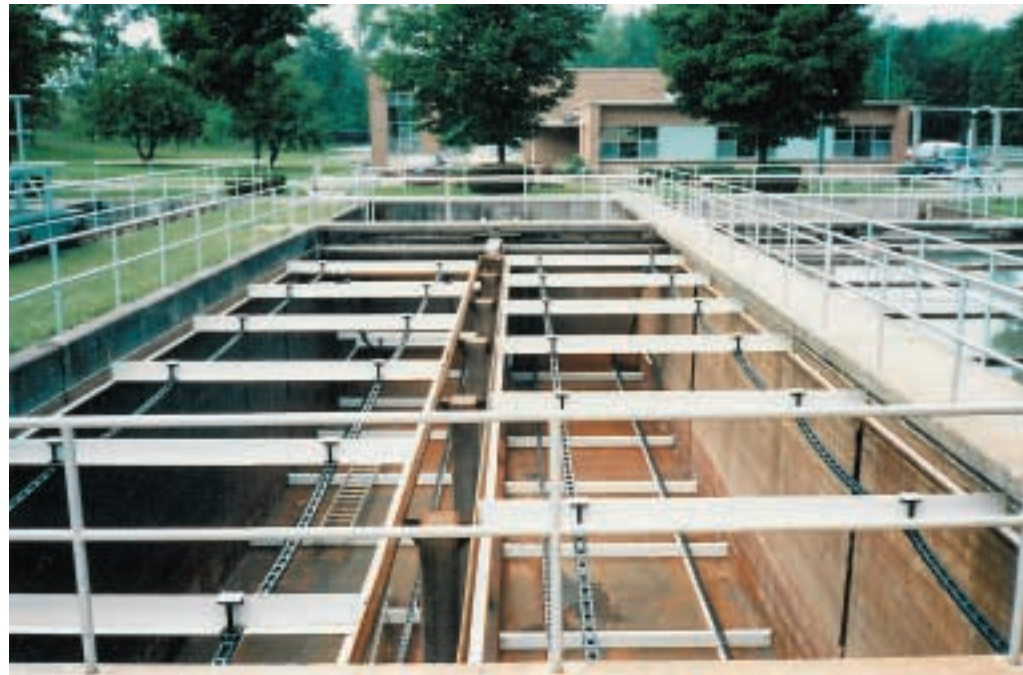
Rectangular Clarifiers During Re Chain
